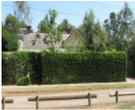
H027 Former Police Station 2.JPG
