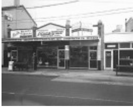
2021a - Brimbank City Council Post-contact Cultural Heritage Study 1998
