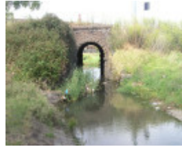
HO41 Railway Culvert 1.JPG
