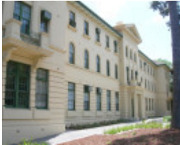
FORMER VICTORIA POLICE DEPOT SOHE 2008
