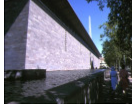
1 national gallery of victoria st kilda road melbourne front view
