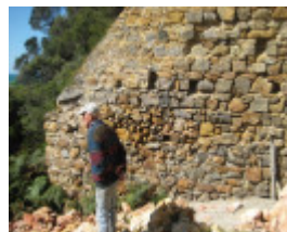
Bell Point Lime Kiln, September 2011
