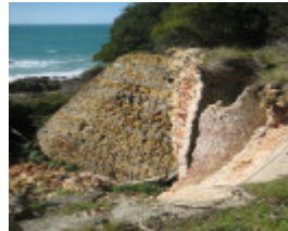
Bell Point Lime Kiln, September 2011
