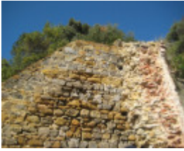
Bell Point Lime Kiln, September 2011
