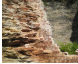
Bell Point Lime Kiln, September 2011
