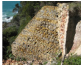
Bell Point Lime Kiln, September 2011
