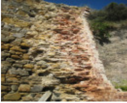
Bell Point Lime Kiln, September 2011
