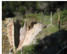
Bell Point Lime Kiln, September 2011
