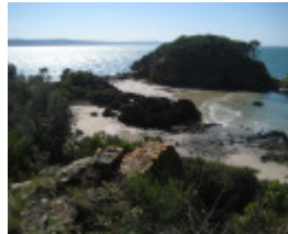
Bell Point Lime Kiln, September 2011
