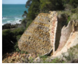
Bell Point Lime Kiln, September 2011
