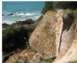
Bell Point Lime Kiln, September 2011
