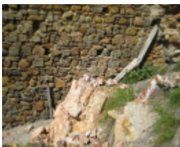
Bell Point Lime Kiln, September 2011
