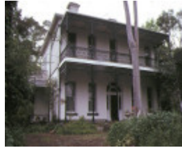
1 barwon cromwell road south yarra front view
