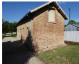
After Photograph - Reference F3879 2016
