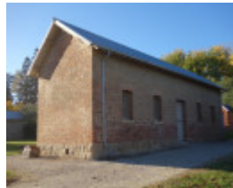
Before Photograph - Reference F3879 2014
