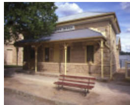
Lands Office Ford Street Beechworth Front View December 1984
