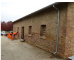
During Photograph - Reference F3879 2015
