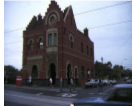
1 former south yarra post office south yarra front view
