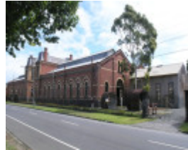
SEWERAGE PUMPING STATION SOHE 2008
