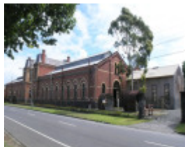
SEWERAGE PUMPING STATION SOHE 2008
