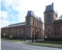
SEWERAGE PUMPING STATION SOHE 2008
