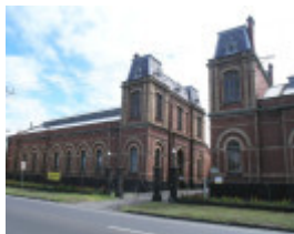
SEWERAGE PUMPING STATION SOHE 2008
