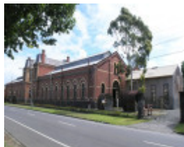
SEWERAGE PUMPING STATION SOHE 2008
