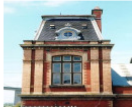
1 former mmbw pumping station douglas parade spotswood tower view aug1987
