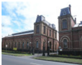
SEWERAGE PUMPING STATION SOHE 2008
