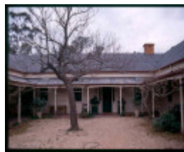
H0305 Tottington Homestead courtyard
