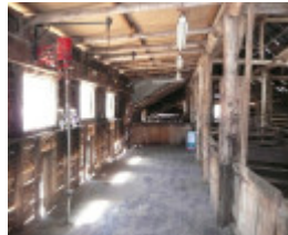
TOTTINGTON HOMESTEAD, STONE COTTAGE AND WOOLSHED SOHE 2008
