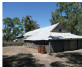
TOTTINGTON HOMESTEAD, STONE COTTAGE AND WOOLSHED SOHE 2008
