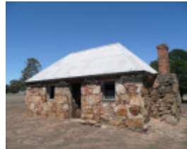
TOTTINGTON HOMESTEAD, STONE COTTAGE AND WOOLSHED SOHE 2008
