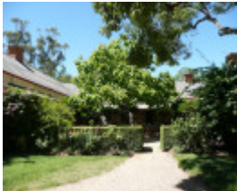
TOTTINGTON HOMESTEAD, STONE COTTAGE AND WOOLSHED SOHE 2008
