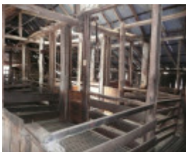
TOTTINGTON HOMESTEAD, STONE COTTAGE AND WOOLSHED SOHE 2008
