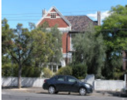
FORMER PRIORY LADIES SCHOOL SOHE 2008
