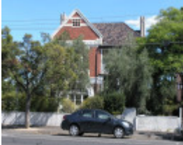
FORMER PRIORY LADIES SCHOOL SOHE 2008
