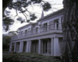
1 oberwyl burnett street st kilda view of balcony & amp; columns
