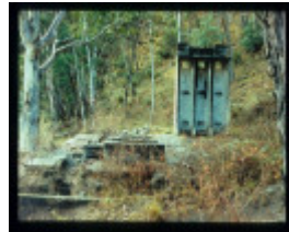
VICTORIA FALLS HYDRO-ELECTRIC POWER STATION
