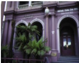
biltmore bridport street albert park front entrance
