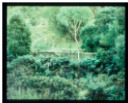
CASSILIS GOLD MINING COMPANY TREATMENT WORKS
