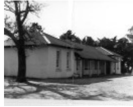
Administration Building, Lake Tyres Aboriginal Mission
