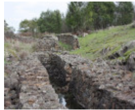
Partial collapse of Bessiebelle July 2013
