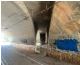
2024. Seam between the 2004 bridge (left) and 1902 bridge (right) viewed from underneath.
