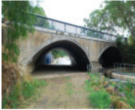
KINGS BRIDGE, OVER BENDIGO CREEK SOHE 2008
