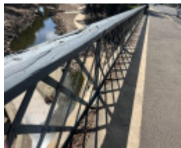
2024. Lattice balustrade, which was relocated to the northern (upstream) edge of the bridge during the bridge extension in 2004.
