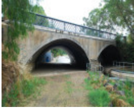
KINGS BRIDGE, OVER BENDIGO CREEK SOHE 2008
