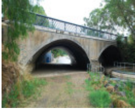
KINGS BRIDGE, OVER BENDIGO CREEK SOHE 2008
