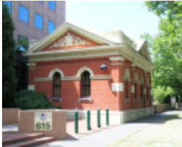
FORMER GAS VALVE HOUSE SOHE 2008
