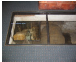
h00675 former gas valve house st kilda road st kilda gas valve she project 2004
