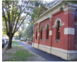
h00675 former gas valve house st kilda road st kilda along street she project 2004
