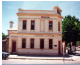
former bank of nsw beechworth front view 1995
