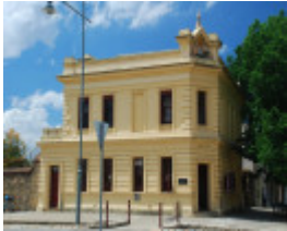
BEECHWORTH WINE CENTRE SOHE 2008
