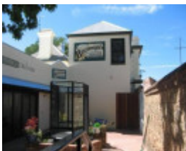
Former Bank of NSW 18 Nov 2014 (25) rear addition
