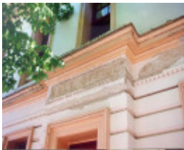
former bank of nsw beechworth facade detail 1995
