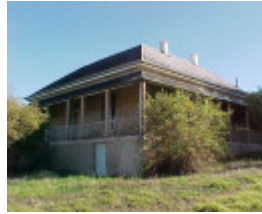
Ledcourt Exterior View May 2001
