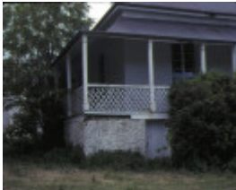
Ledcourt Homestead Stawell Verandah View May 2001
