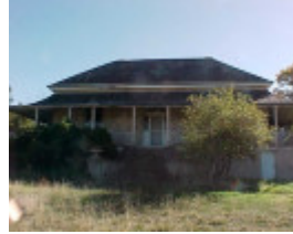
Ledcourt Exterior Entrance View May 2001
