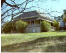
1 ledcourt homestead exterior front view may2001
