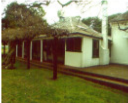
1 killeen homestead with verandah august2000.jpg
