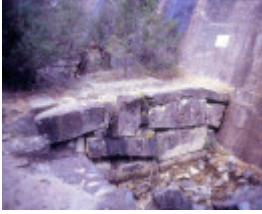
h01556 heatherlie quarry grampians national park halls gapp rock and concrete crane base she project 2004
