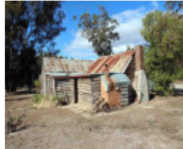
Masters House west side (Peter Mills photo 2642013).jpg
