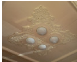
Horsham Theatre detail of ceiling 2009
