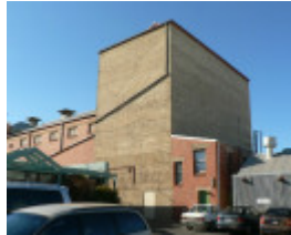
Horsham Theatre rear view of fly tower 2009
