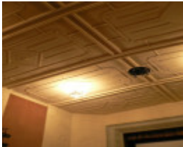
Horsham Theatre detail of auditorium ceiling 2009
