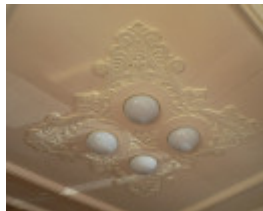
Horsham Theatre detail of ceiling 2009
