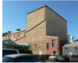
Horsham Theatre rear view of fly tower 2009
