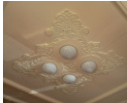
Horsham Theatre detail of ceiling 2009
