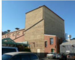
Horsham Theatre rear view of fly tower 2009
