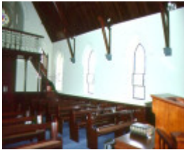
St Johns Streatham Interior September 2000
