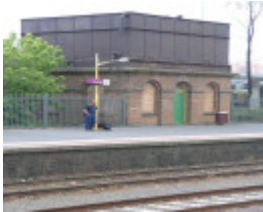
WATER TOWER SOHE 2008
