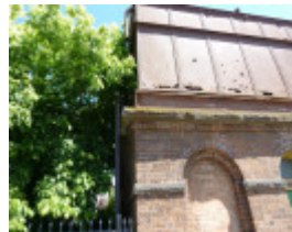
H1673 WATER TOWER LHA 2015 3.JPG
