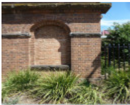
H1673 WATER TOWER LHA 2015 2.JPG
