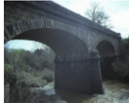
1 bridge over jackson's creek sunbury side view sep1984
