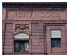
11447 Northcote Cinema 212 220 High Street Facade Detail 2 31
