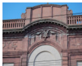
11447 Northcote Cinema 212 220 High Street Facade Detail 1 31
