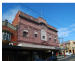
11447 Northcote Cinema 212 220 High Street View South East 31
