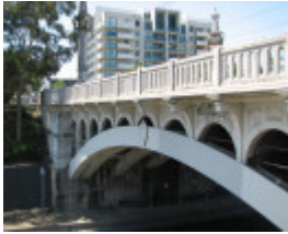
CHURCH STREET BRIDGE SOHE 2008
