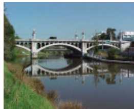
1 church street bridge from se bank mar01
