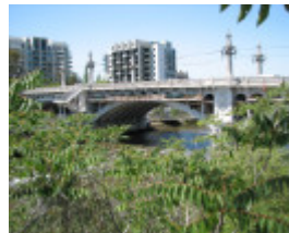
CHURCH STREET BRIDGE SOHE 2008
