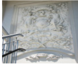
CHURCH STREET BRIDGE SOHE 2008
