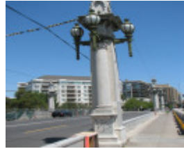
CHURCH STREET BRIDGE SOHE 2008
