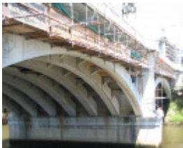
CHURCH STREET BRIDGE SOHE 2008
