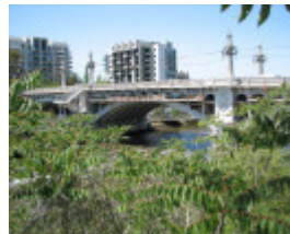
CHURCH STREET BRIDGE SOHE 2008
