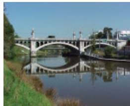
1 church street bridge from se bank mar01
