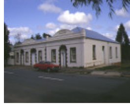
1 tarnagulla public hall commercial road front view sep1992
