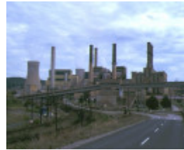
1 yallourn a b c d & e power stations latrobe valley yallourn property view
