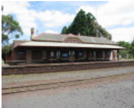
Terang RWS Station Building Platform February 2002
