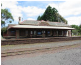
Terang RWS Station Building Platform February 2002
