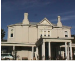
Cooring Yering House
