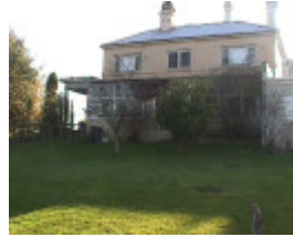
Cooring Yering House
