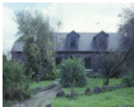
1 graffs farm thomas street thomastown front view
