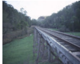
rail bridge curdies river timboon rail tracks jun1984
