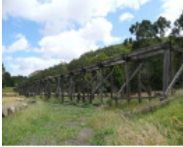
RAIL BRIDGE SOHE 2008
