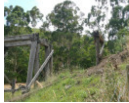
RAIL BRIDGE SOHE 2008
