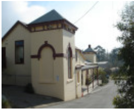
Former Cheese & Bacon Curing Factory
