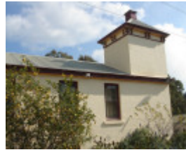
Former Cheese & Bacon Curing Factory
