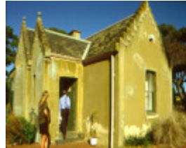
1 overnewton gatehouse h1947 march 2001
