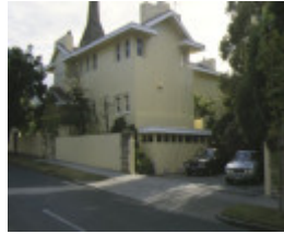
1 clendon lodge clendon rd toorak view from street feb1986
