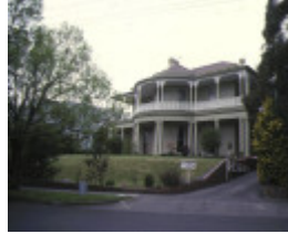
1 trawalla lascelles avenue toorak front detail
