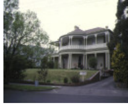
1 trawalla lascelles avenue toorak front detail
