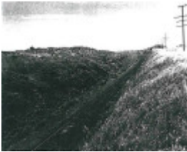
Ingliston Bank railway cutting and piles of remnant railway
