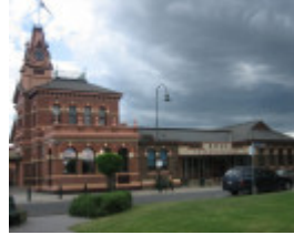
Traralgon Post Office from the north side
