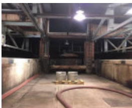
2019 wine press in cellar.jpg
