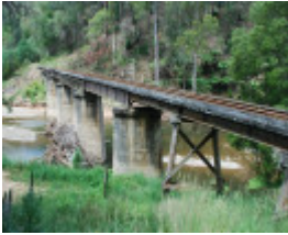
RAIL BRIDGE SOHE 2008
