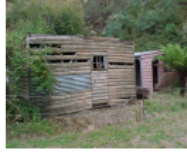
Walhalla Post Office Exterior Outbuildings March 2003
