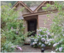
Walhalla Post Office Exterior Twin Gables March 2003
