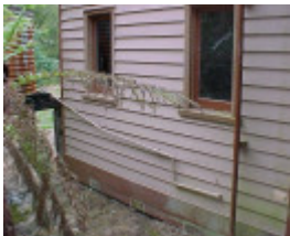
H00583 walhalla po exterior openings mar 2003
