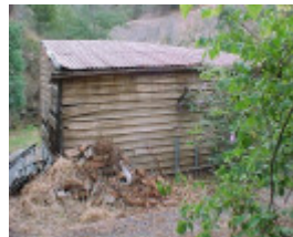
H00583 walhalla po exterior outbuilding mar 2003
