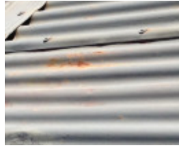
Before Photograph - Reference F3834 2014
