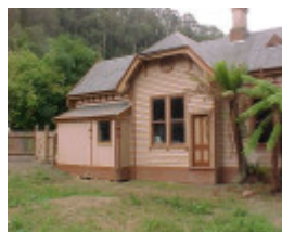
H00583 walhalla po exterior3 mar 2003
