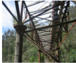
Brunton s Bridge from below
