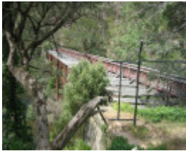
Bruntons Bridge Thompson River
