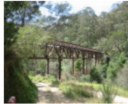
Bruntons Bridge Thompson River, 2006
