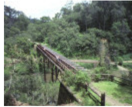
1 bruntons bridge thomson river narracan front view 1983
