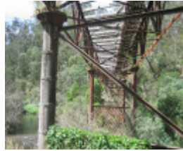
Bruntons Bridge Thompson River
