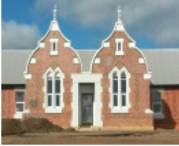
Main facade in July 2018
