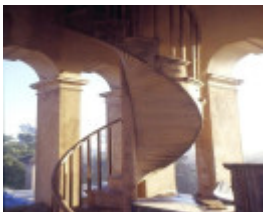
bontharambo homestead boorhaman road wangeratta spiral staircase in tower she project 2003
