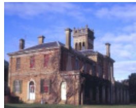
bontharambo homestead boorhaman road wangeratta back view of homestead she project 2003
