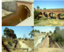
1 main outfall sewer collage
