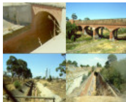
1 main outfall sewer collage
