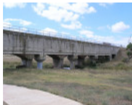
MAIN OUTFALL SEWER SOHE 2008
