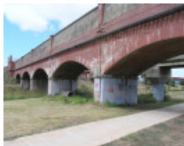
MAIN OUTFALL SEWER SOHE 2008
