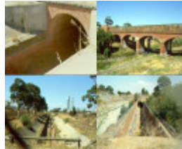
1 main outfall sewer collage
